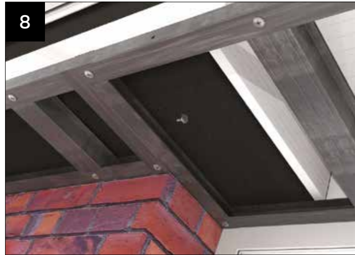
Screw split horizontal frames together using CHAA006 (bag of 25).
