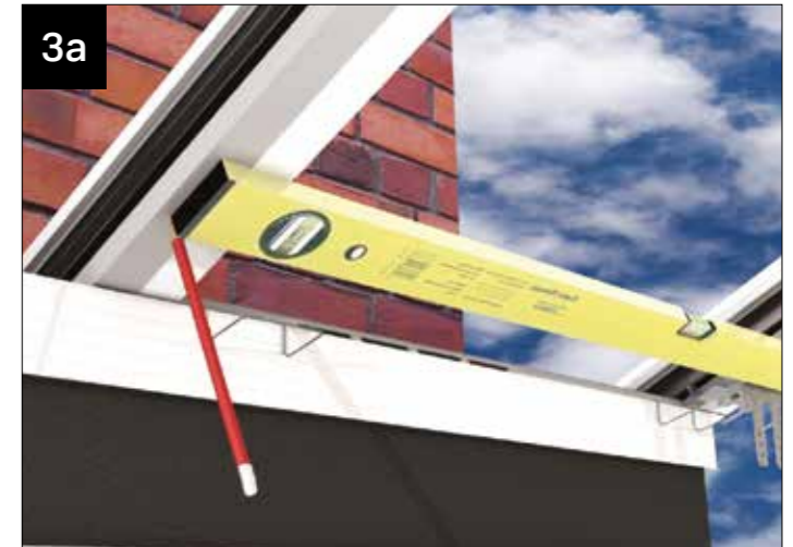
FITTER TIP: If possible, check and line through with the bracket position on the adjacent full length bar. Mark the bracket positions on the bars of the box gutter.
