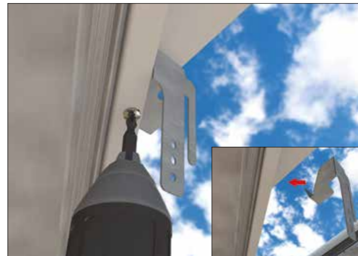
NOTE: The transom bracket CHAB001 MUST be trimmed and adapted to suit situations where a transom bar, valley and internal insulated pelmet vertical frame intercept, as shown above.
