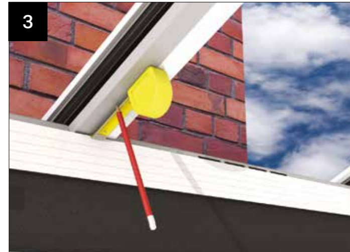
Using LHE---/2 as a datum, measure and mark the positions of the brackets in line with the dimensions given in the provided paperwork.
